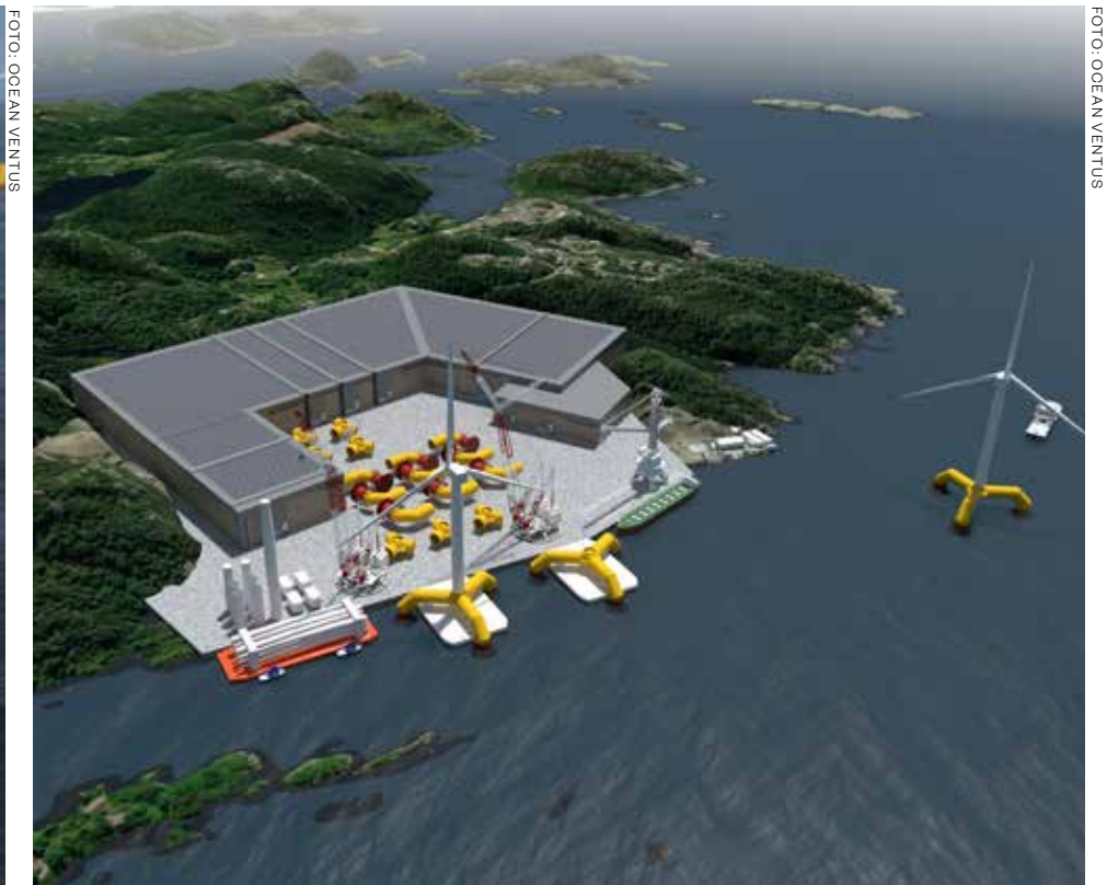
The Ocean Ventus prefab factory for FOWT substructures
