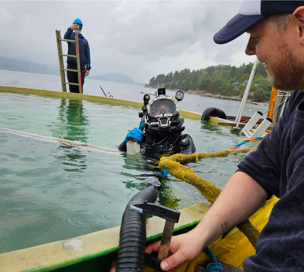
Figure 0-2 Falck Dykk, Submara preparing for ex-situ IWC procedure in WST2 tank at NIVA Solberstrand in 2025. Source NIVA.
